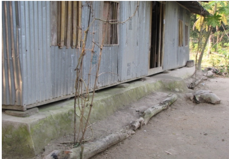
Photo 1: Floating pillar of a House
